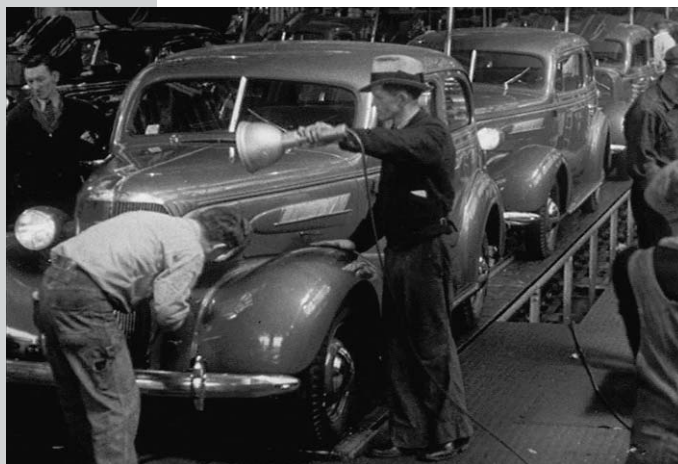
Chevrolet Motor Company's Master Hands (1936) traces the manufacture of an automobile from foundry to finished product. Industrial films such as this documentary short will be covered in an NFPF guide slated for publication in 2006.
